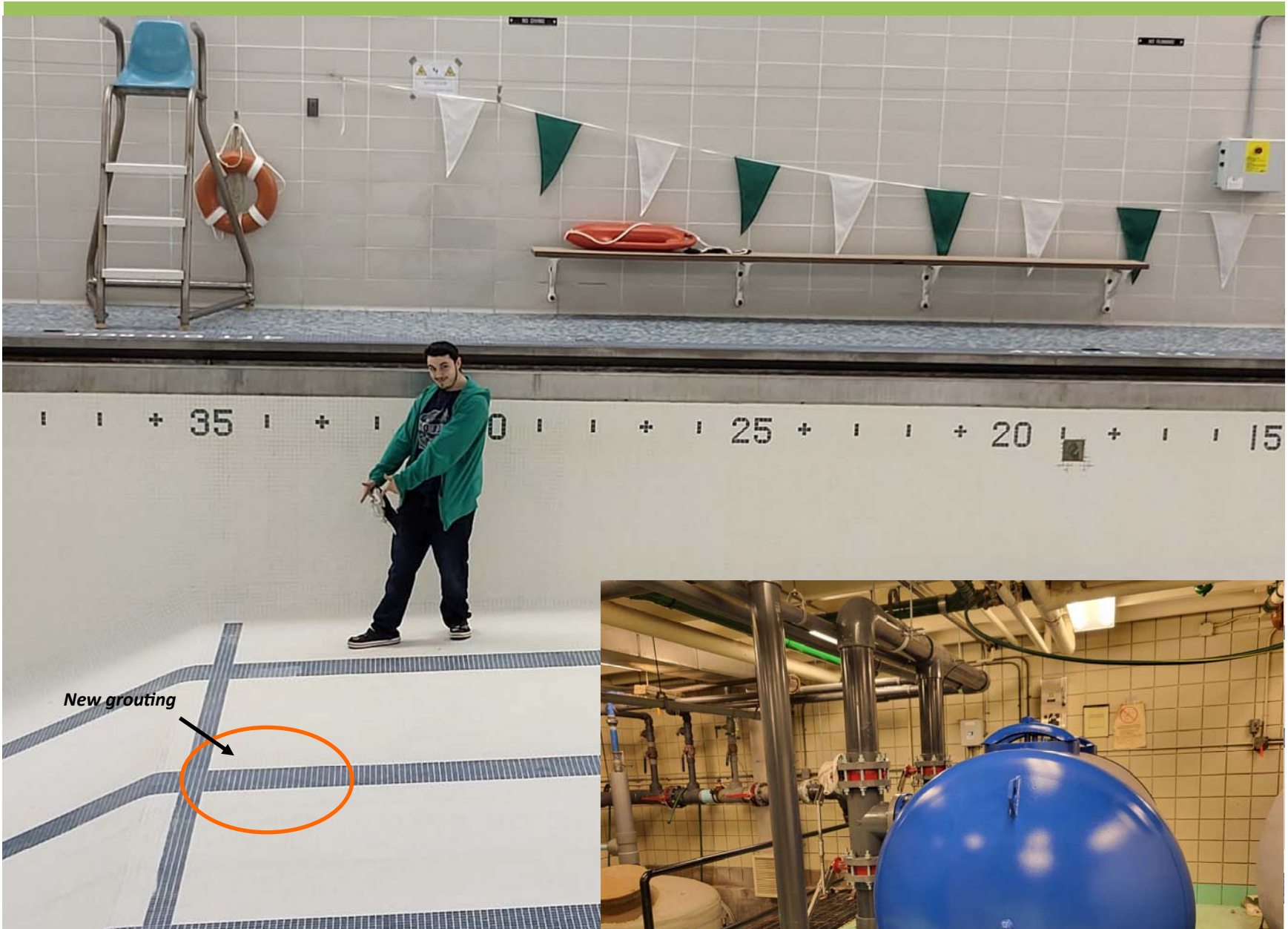
Above: Ryan Bruer points out one of the sections of the Middle School pool that Scott Cameron regouted this summer. Right: The new filtration tank at the Middle School filters 400 gallons of water per minute from the 166,000 gallon pool.
